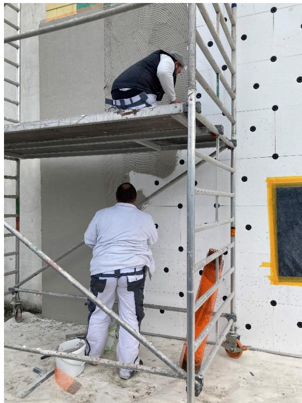
Figure 23: Application of the base coat layer
