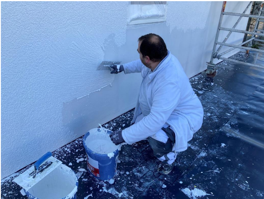
Figure 27: Application of the top coat
