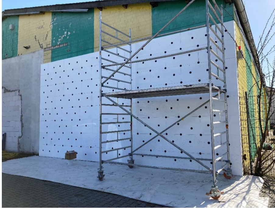
Figure 22: Test façade fixed with anchors
