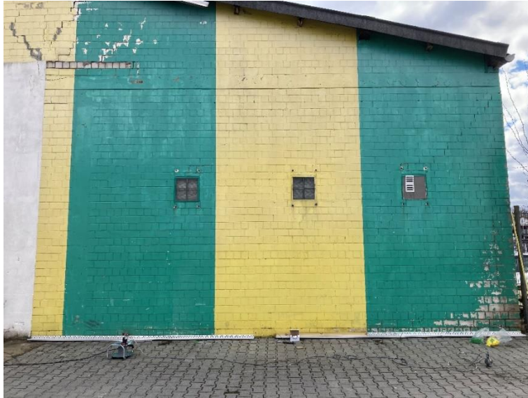
Figure 17: CREAToR test façade in its original state
