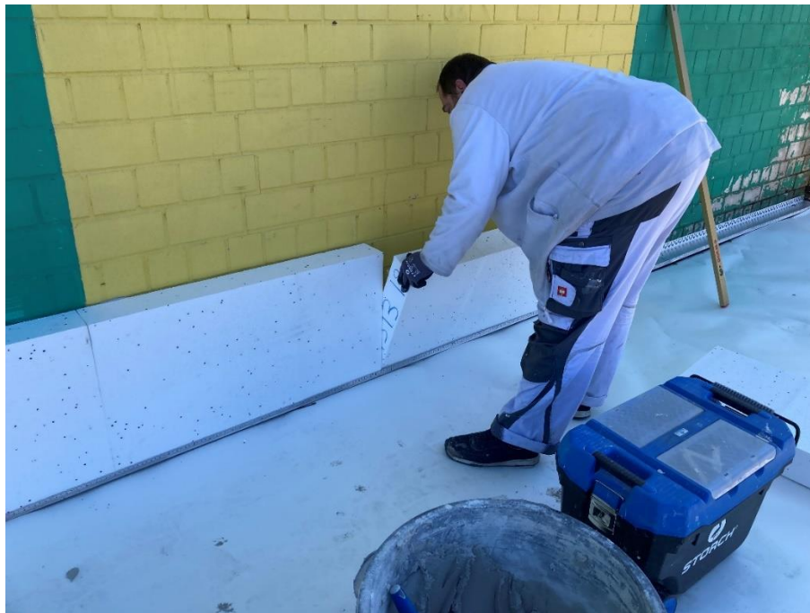
Figure 19: Attaching the EPS board to the wall
