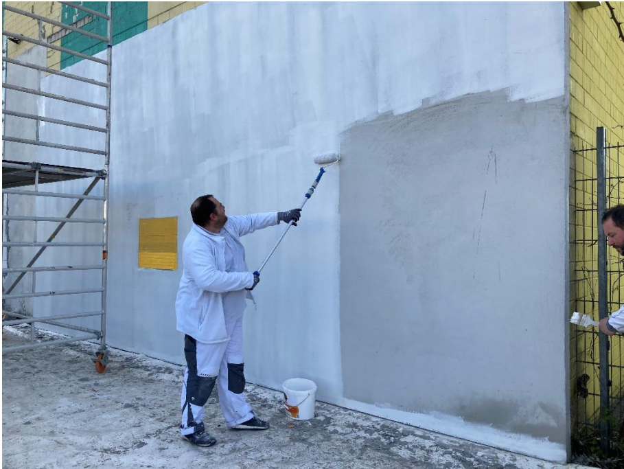
Figure 26: Application of the primer coat
