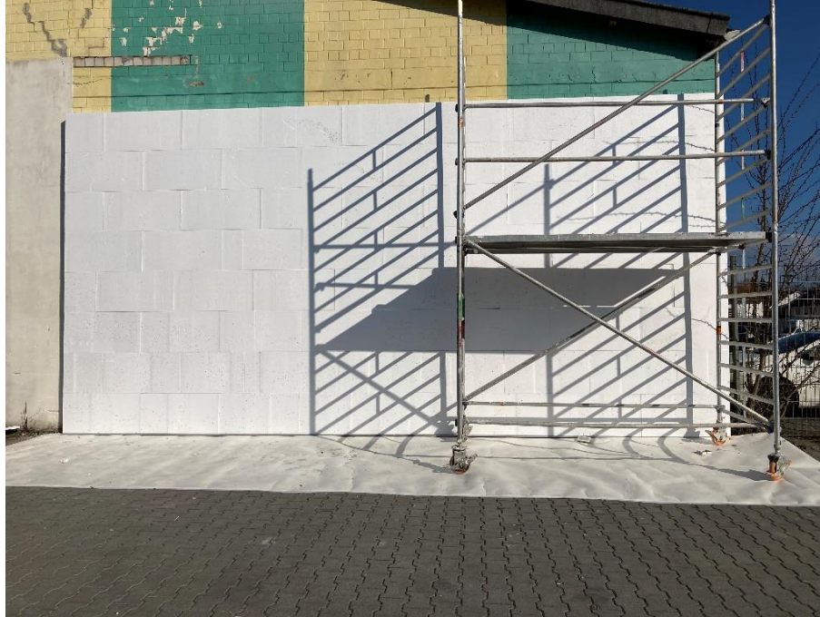
Figure 20: CREAToR test façade with attached EPS boards
