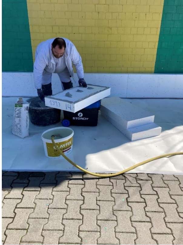
Figure 18: Application of adhesive on CREAToR EPS thermal insulation board
